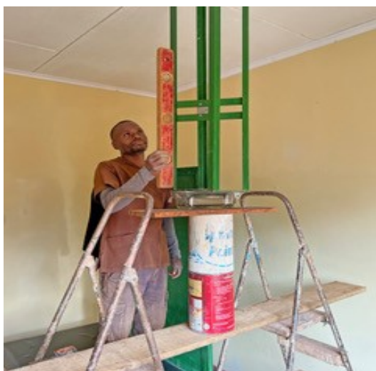
Mounting of x-ray-tube support, making sure it is vertical
